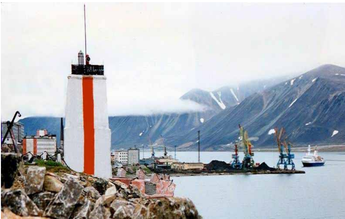
Figure 6: The laser leading beacon collocation on the front structure of the Lihachyvsii leading range of Providence Bay
